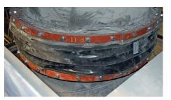
Existing steel parts were re-used in most of expansion joints.
